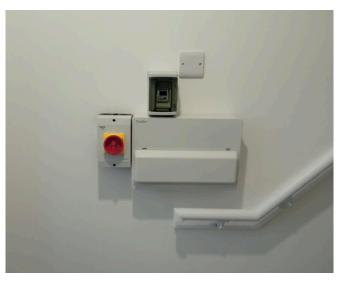
There is an isolator for the PV panels located in the hallway, please only use this in a case of emergency.
