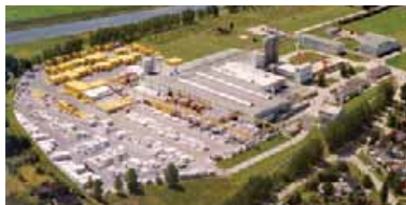
Calbe Factory, Germany
