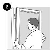
Lift the door leaf off the hinges from the frame and store safely. Note: If a head fixing brake is installed, unscrew and remove prior to lifting the door.
