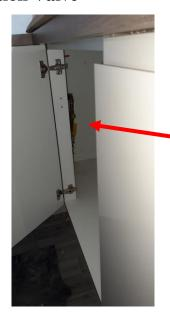
Your gas supply can also be turned off at the yellow handle isolation valve which is in the kitchen cupboard underneath the sink
