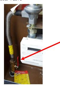
Your gas supply can also be turned off at the red handle isolation valve which is in the Brown Meter Unit on the outside wall
